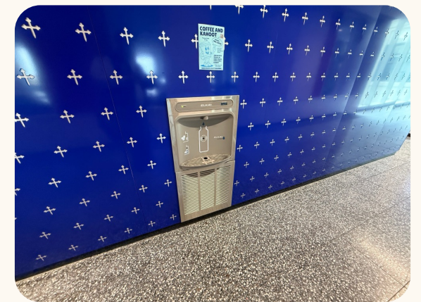
PHOTO: Water fountain
