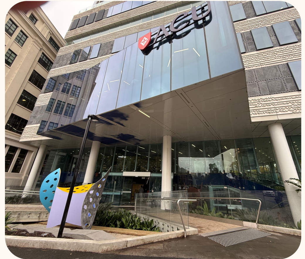
PHOTO: Building exterior from Victoria Parade
